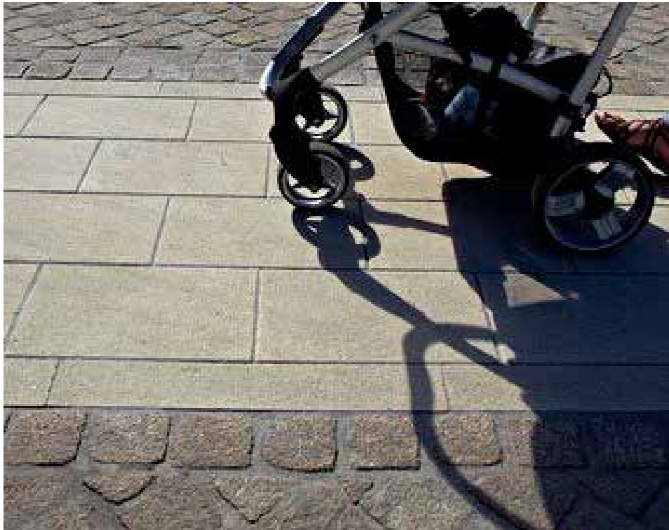
Above: mix of permeable pre-cast paving elements ('Clima-Pave Grange' by Kilsaran) and stone sett paving to Home Zone area
